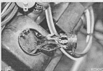
Repair of the rectifier tube socket
